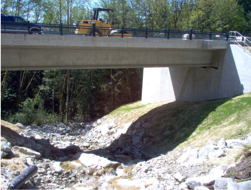
Marr Creek Bridge – British Properties West Vancouver
