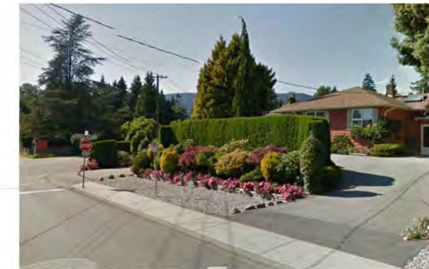
Existing house to the North
