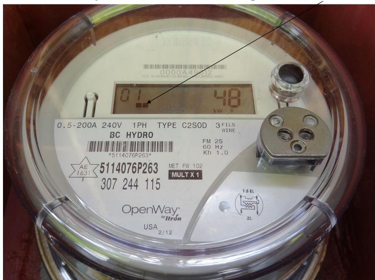
Each "pulse" represents the consumption of 1Watt-hr A display, comprised of 2 squares and > triangle.
