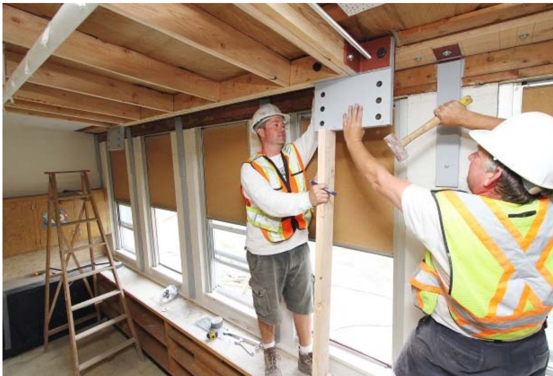
Workers install wall improvements at Mckenzie elementary school in Victoria in July, 2011, as part of seismic upgrades to the school.
