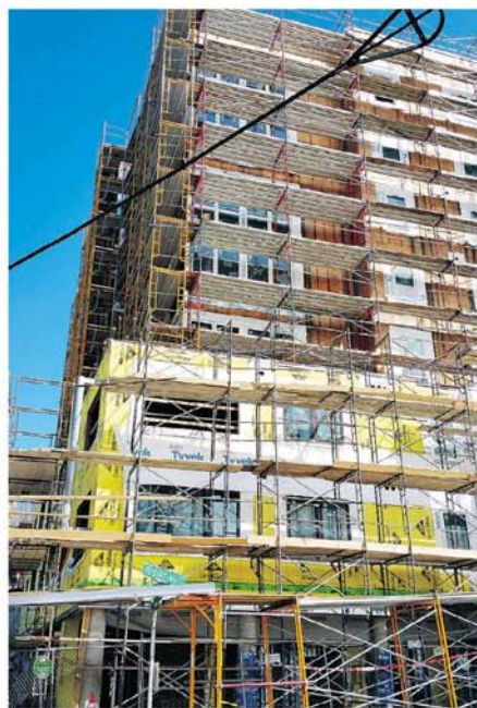
This cost-effective form of medium-rise public housing in a Seattle mixed-income neighbourhood, combines five storeys of wood-frame construction above three levels of concrete construction.
