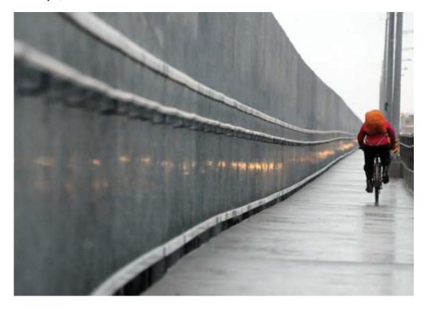
A cyclist heads south on the newly opened east sidewalk of the Ironworkers Memorial Second Narrows Crossing. After more than a year of construction, the sidewalk is now twice as wide with a new safety barrier. The west sidewalk is expected to remain closed until the fall of 2015 while it is widened. Photo Mike Wakefield
