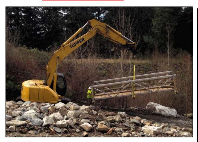
**TRAIL FIX** District of North Vancouver workers lower a new bridge across Mackay Creek near the base of Grouse Mountain Jan. 21. The bridge on Upper Powerline Trail was damaged by debris during heavy rainfall in November. The district pegs the total cost for area remediation, debris removal and bridge construction at \$100,000. The trail was reopened last week.
