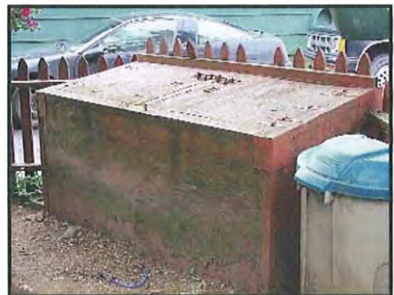
Side view of the enclosure pictured on the left with metal flashing on seams and seamless construction.
