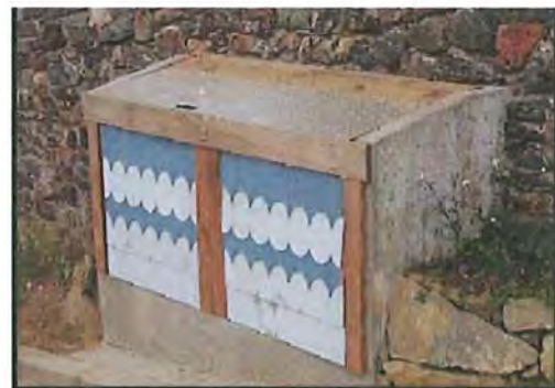
Concrete enclosure. Cement sides and base, steel top, and seamless construction.
