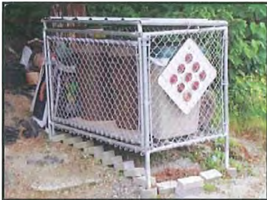
Chain link enclosure - this one would be more secure without the gaps above the front door and near the top. Strengths: Has roof cover to shed rain and snow. Anchored to ground. Weaknesses: Lots of places for claws to grab and pull. Cans visible to bears.
