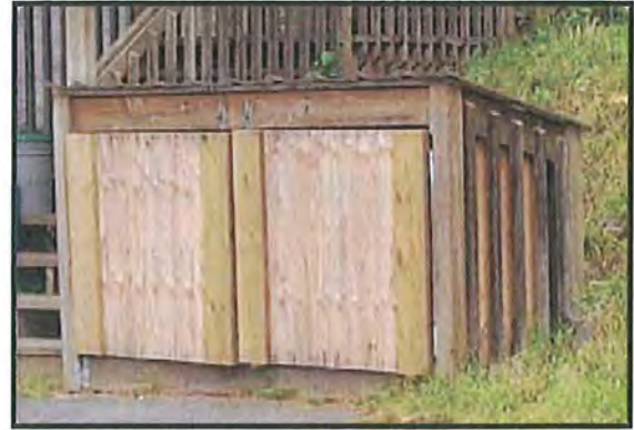
Wooden enclosure. Strengths: Secured to ground and stairs. Weaknesses: Seams too big, claws can grip, sides can be pulled off. Roof has visible seam and may be torn off.
