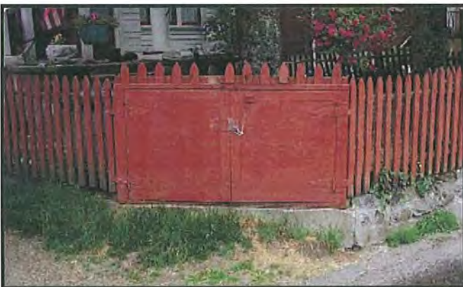
Wooden enclosure. Strengths: Secure to ground, seamless construction, directly accessible to refuse collection, and clip fastening latch.
