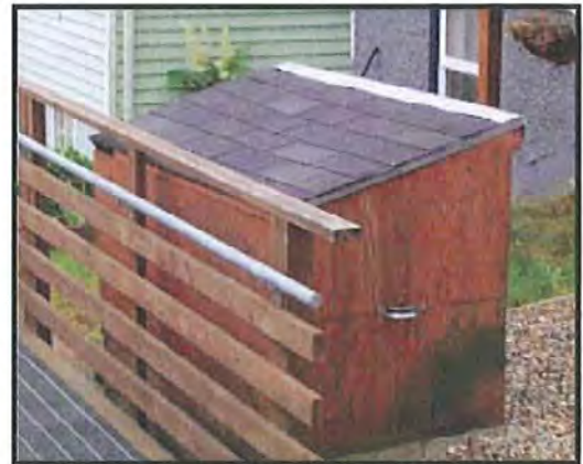
Wooden enclosure. Strengths: Seamless construction, metal flashing on seams, and minimal overhang of roof.
