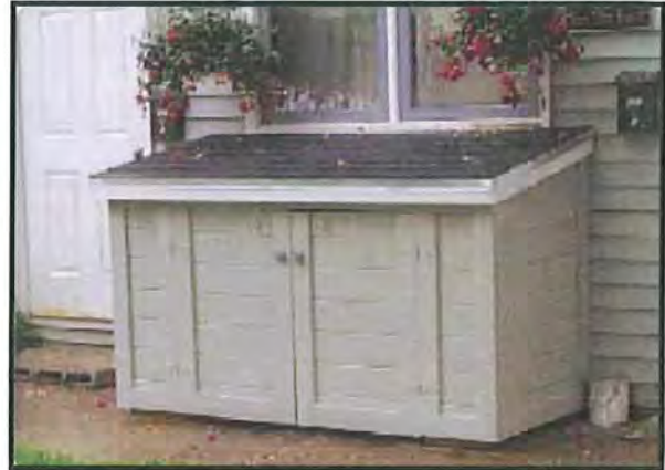
Attractive enclosure with pitched roof to shed snow. Strengths: Minimal seams. Weaknesses: Hinges and latches not heavy duty.
