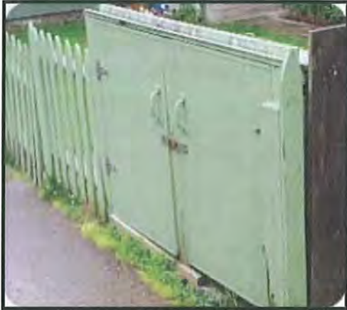
Make sure that the doors fit together snugly with no gaps that bears can get claws into.
