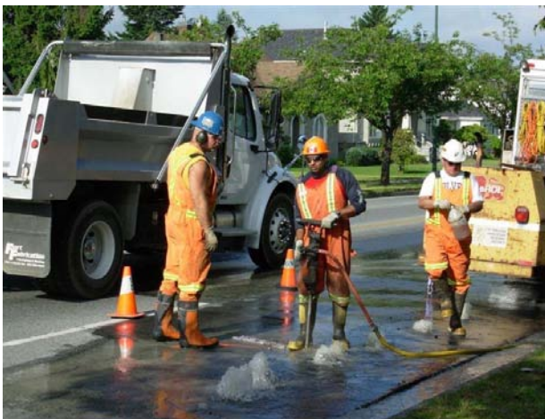
Figure 14: Repairing Watermain Leak
