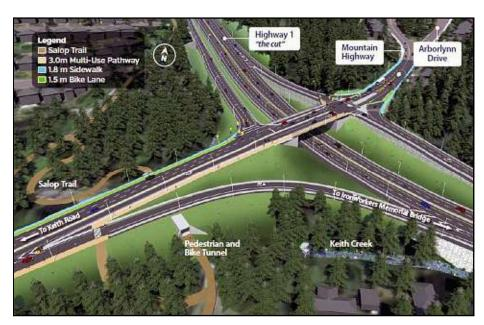
The Highway 1 at Mountain Highway interchange project includes four ramps, a new, wider structure with signalized intersections, and realignment of Mountain Highway to Brooksbank Avenue at Keith Road. IMAGE SUPPLIED
