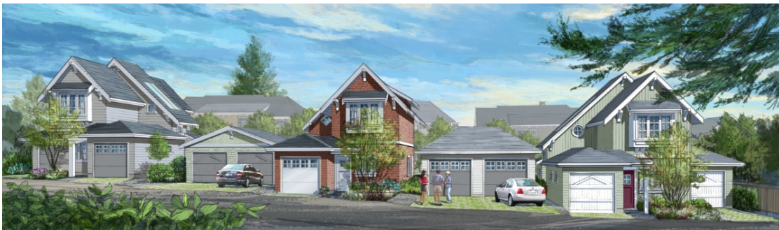
Strata-Titled Coach Houses at “Hollyburn Mews”, West Vancouver (under construction)
