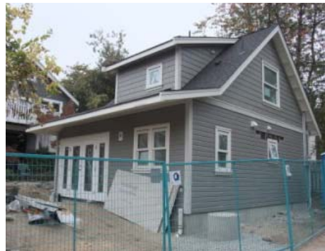
Level ‘B’ Coach House (nearing completion)
