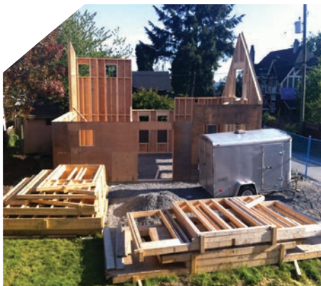
Coach House under construction. Frames are made off-site for faster installation.
