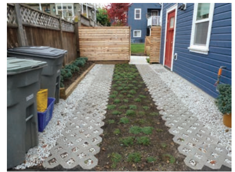
Example of permeable parking treatment
