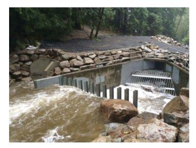
Water gushes through the revamped culvert and grates on Kilmer Creek Saturday. During a bad storm last November, the culvert became blocked with debris and several homes flooded. photo supplied
